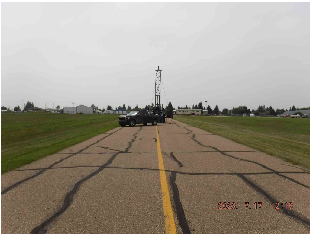
Photograph 6: Looking southwest toward BH23-08
